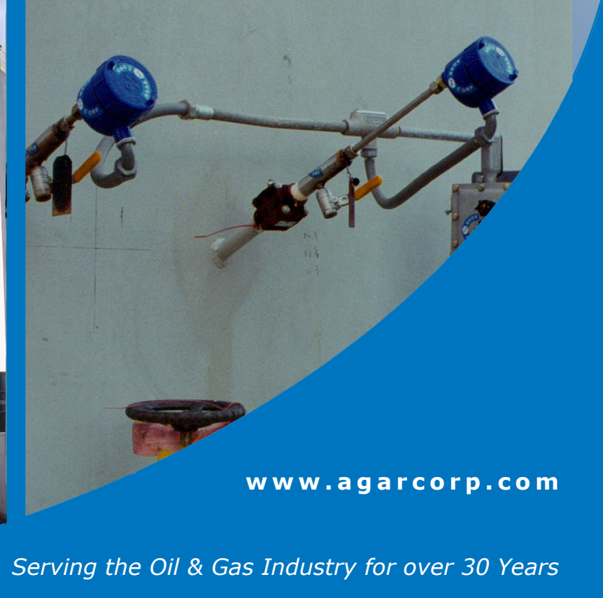
Automatic Tank Dewatering INTERFACE CONTROL
